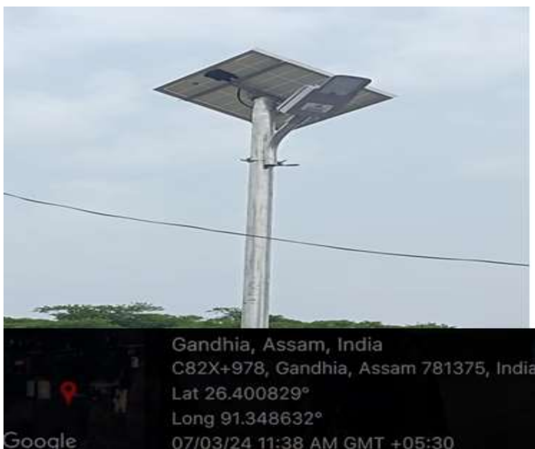
17. Newly installed Solar light
